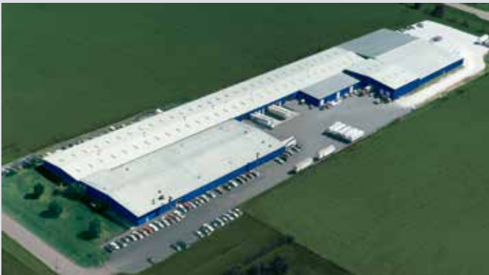
Hörmann LLC, Montgomery, IL Headquarters and Manufacturing Plant
