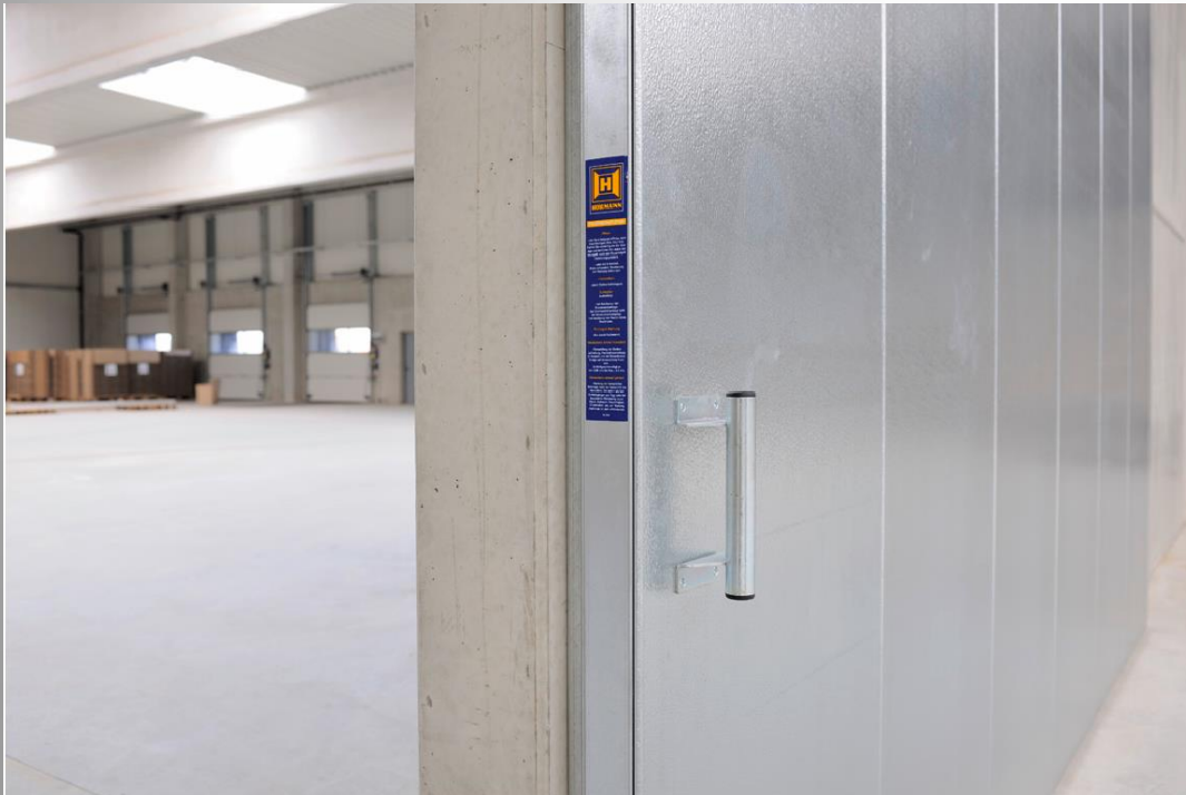
Picture 10: Fire sliding door in a warehouse. Optionally the pearlgain surface can be coated in RAL of your choice
