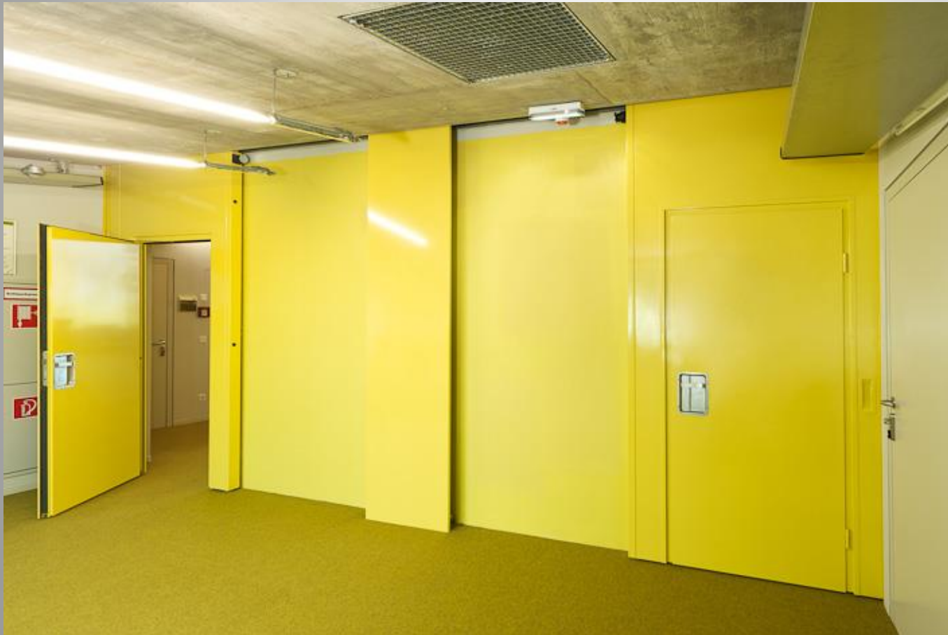
Picture 9: 2 Fire sliding doors with wicket door without threshold
