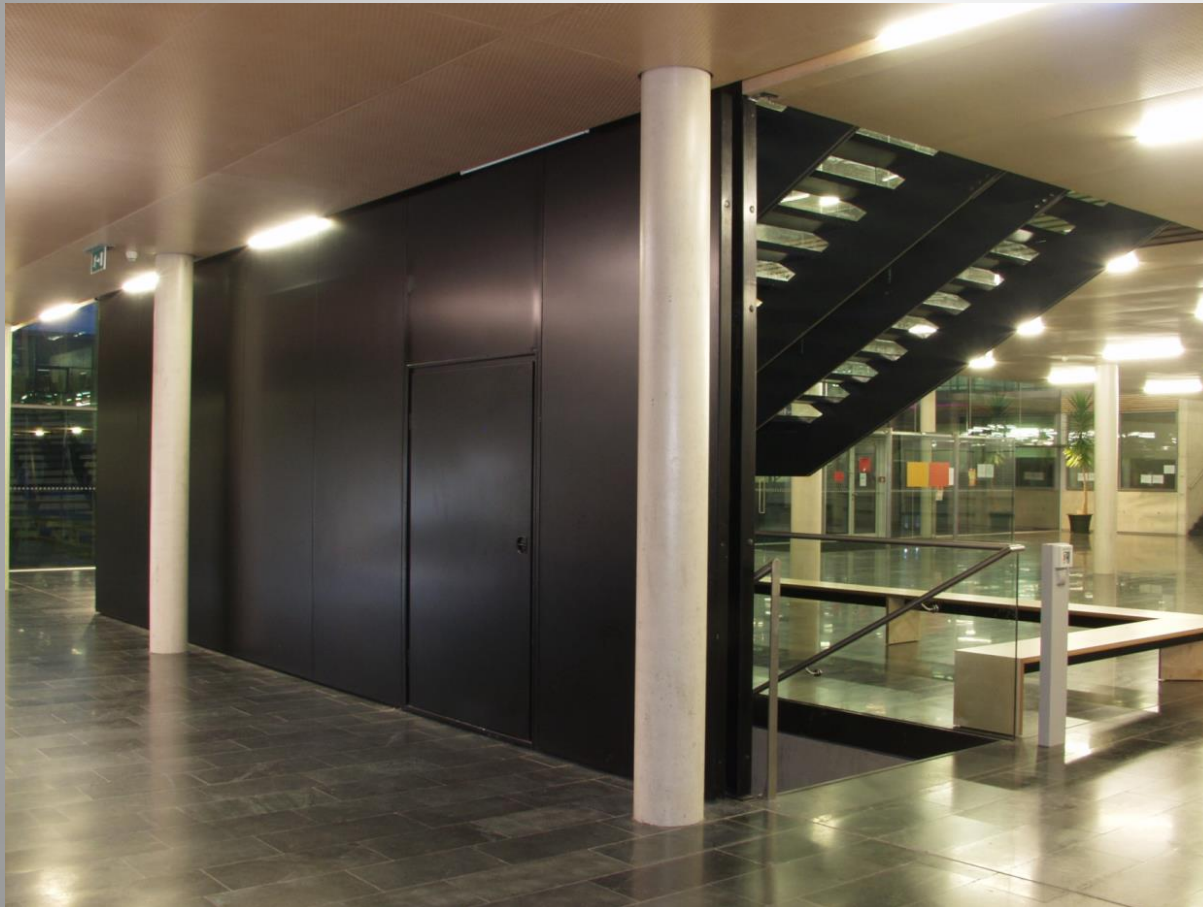
Picture 3: Fire- & smoke- tight sliding door in a school building
