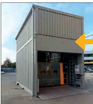
Temporary solution during site refurbishment
