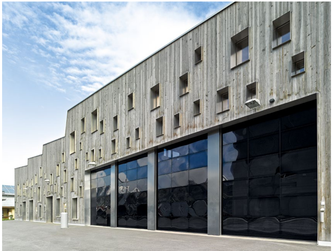
TOP. ALR F42 Vitraplan with grey tinted glazing integrated in the glass facade
