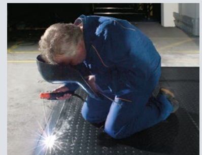
Weld to the edge brackets – done!
