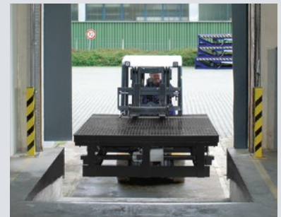
Position the new dock leveller
