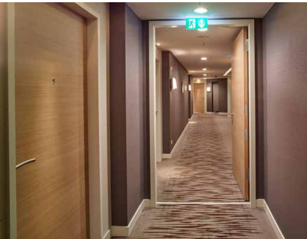
LEFT. Steel frames with high-quality fire-rated doors
