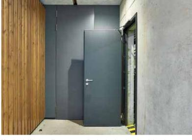
Material mix: Wood panelling, concrete wall and anthracite coloured steel sheet door.
