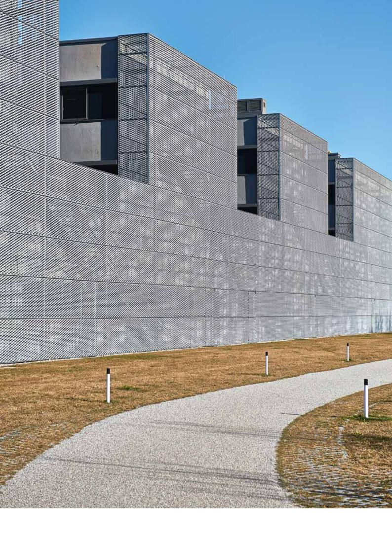
The skin made of expanded metal is spaced 40 to 150 centimetres to the massive building body. (previous page)
