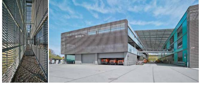
The fleet and storage rooms can be reached from within the covered walkway by means of industrial sectional doors. The inner rooms benefit from light falling into the walkway thanks to the glazing. (top) Up close, the shell made of expanded metal reveals what it's hiding. (bottom left)
