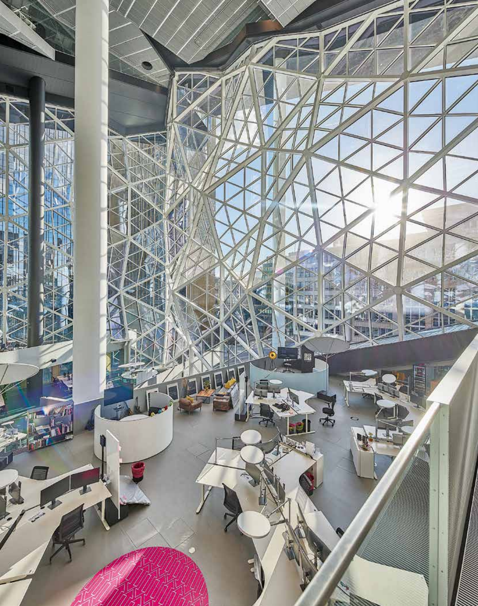
The glass facade lets in a lot of sunlight from the southwest, meaning that staff have to use sunshades for protection.
