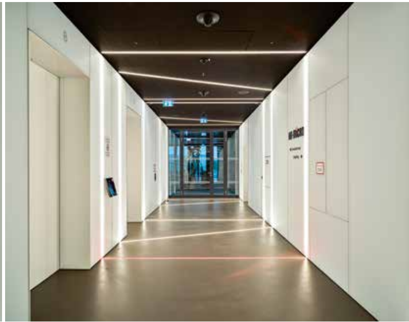
The double-leaf T30 recessed doors with glass overlay are not visible when open – they are integrated flush into the wall.
