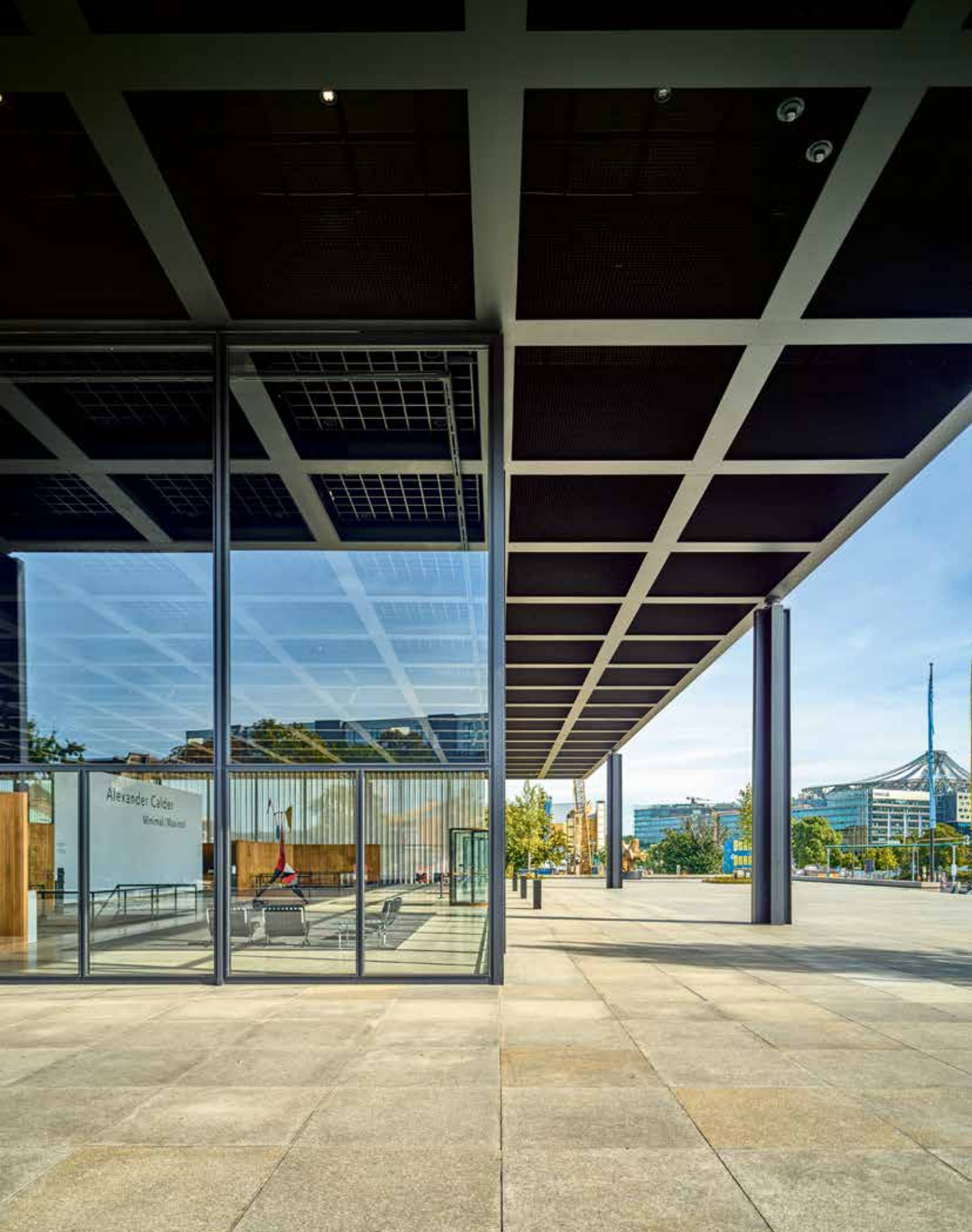
Finally contemporary: The facade is now thermally separated and the panes are made of insulated glass.
