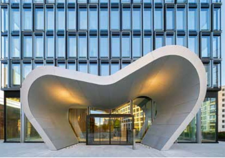
The entrance area clearly stands out against the orthogonal facade.
