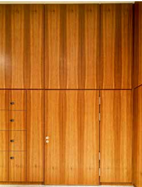
Doubled door to create flush walls.
