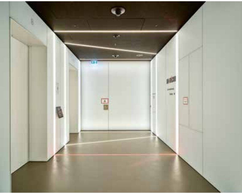
The double-leaf T30 recessed doors with glass overlay are not visible when open – they are integrated flush into the wall.
