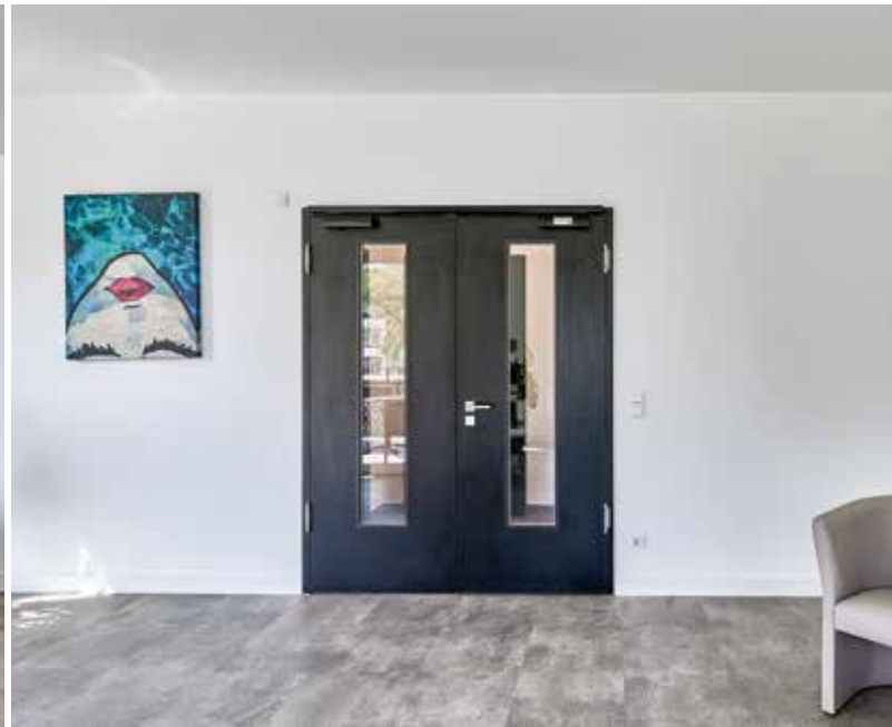
Similar rooms, different look: Schörghuber's double-leaf T30 doors are finished with a white or black HPL laminate.
