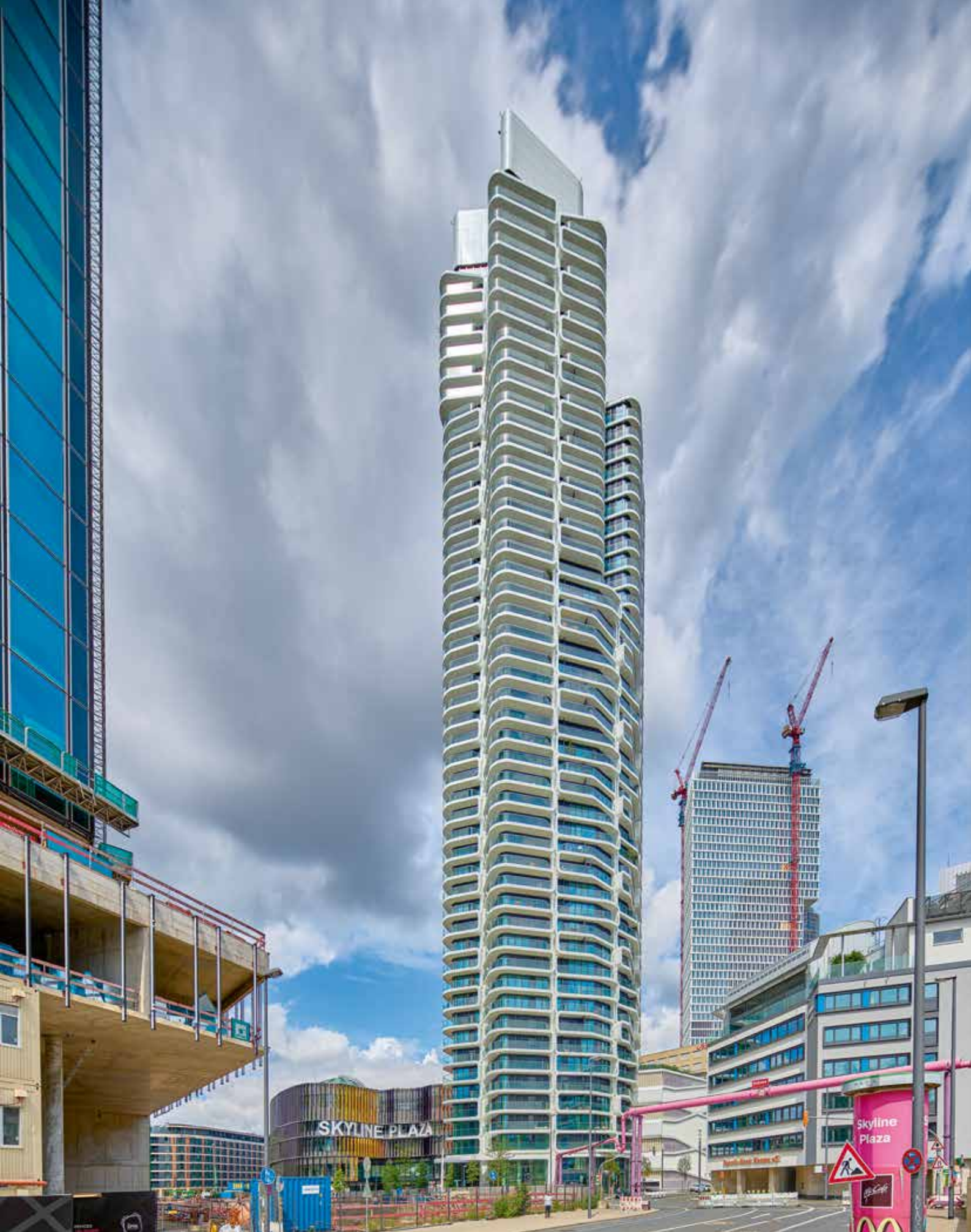
Central location: The Grand Tower with Skyline Plaza in the background – and in the foreground the construction site of Tower One by Meurer Architektur.
