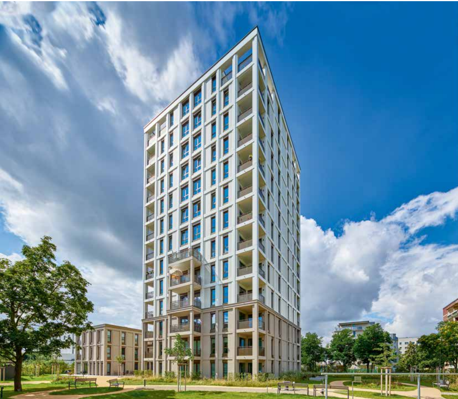
Mullions and transoms can be clearly seen in the facade. The fact that the facade is stepped at different levels gives the building structure.
