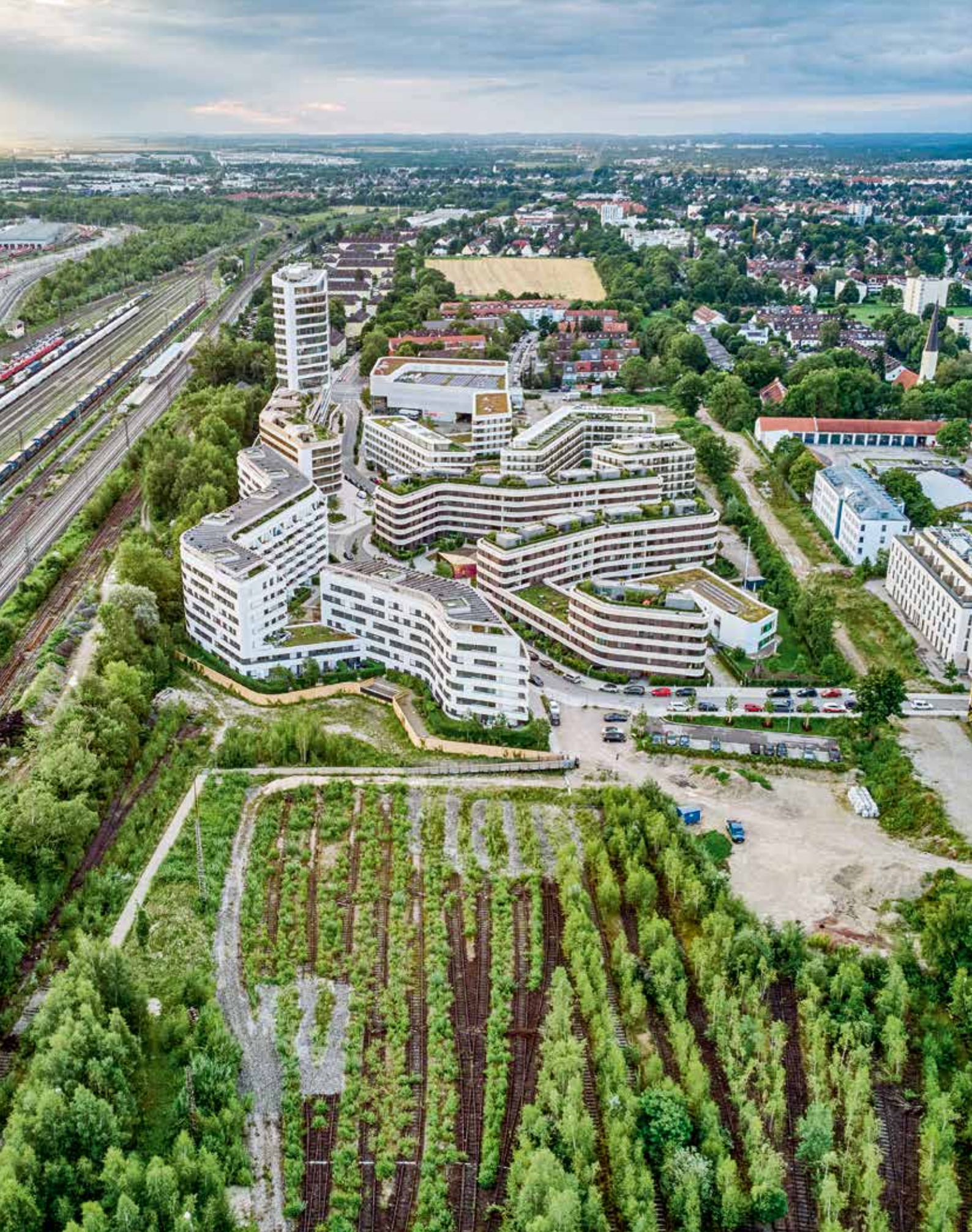
A triad of man-made green spaces: allotment gardens on the left, the overgrown old railway tracks below – and, providing a synthesis, the NEO rooftop garden.
