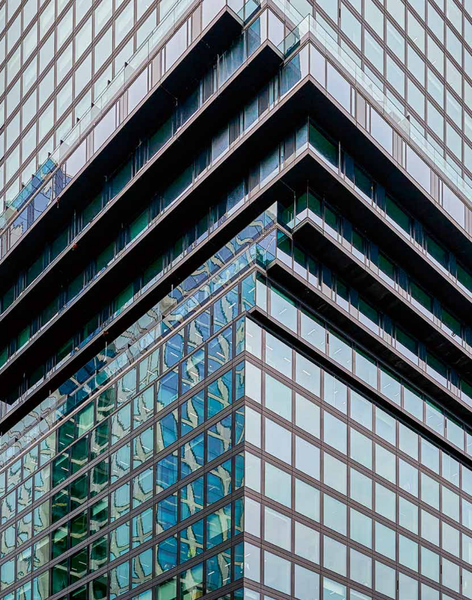
The "hip swing" between floors 15 and 23 clearly indicates where the apartments are located in the Omniturm. It juts out up to four metres.
