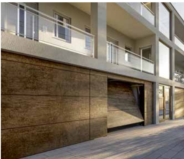
Design accent: collective garage door with Corten steel surface.
