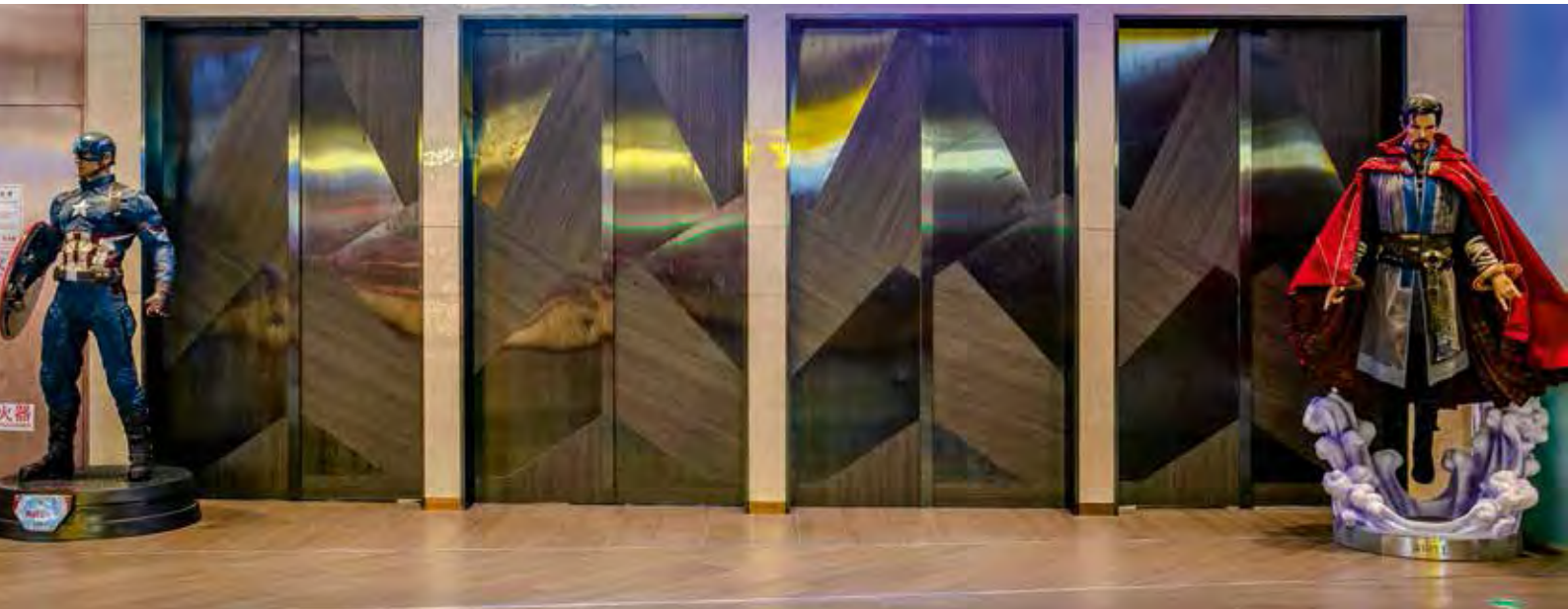
You don't need a superhero to provide safety in the case of a fire. The fire-rated doors at the entrance to the IMAX cinema take over this feat.
