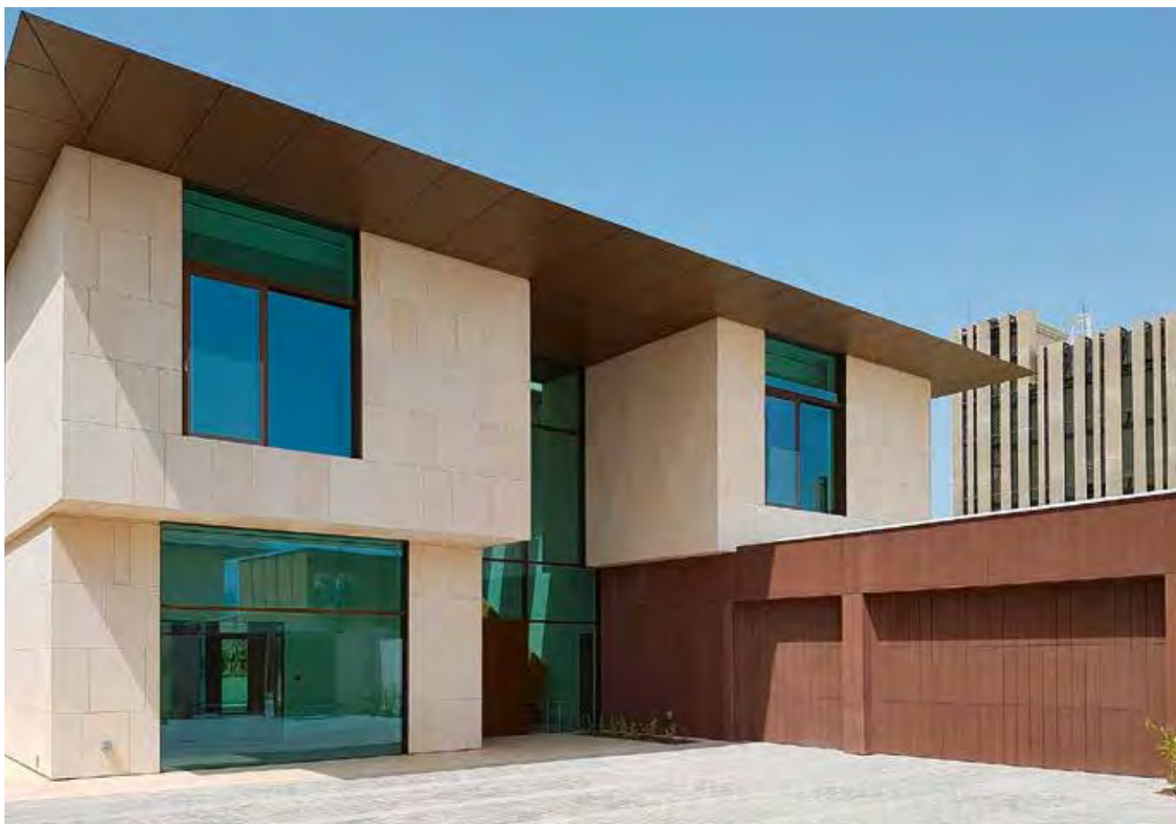
The villas are fitted with ET 500 collective garage doors from Hörmann, clad with the facade material.
