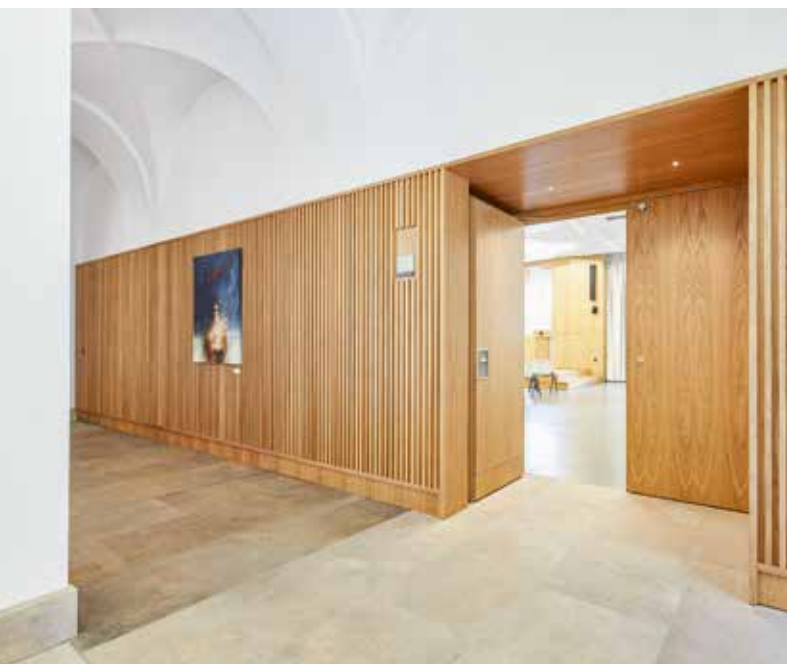
The double-leaf door can be held open by means of magnets.
