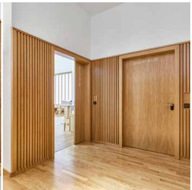
Acoustic-rated doors ensure that there is silence during prayer.
