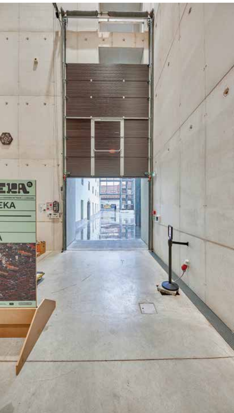
Visible technology: the industrial sectional door with vertical fittings.
