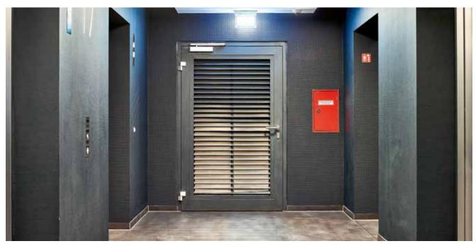
Opaque but not airtight: The custom-made product consists of a Hörmann tubular frame part and a mesh insert from Renson.
