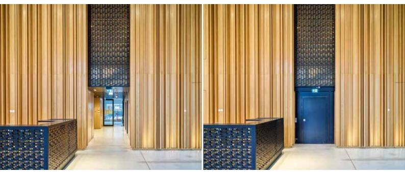
In daily operation, the fire sliding door is invisible. You would only see that it matches the colour of the perforated steel surfaces in the event of a fire.
