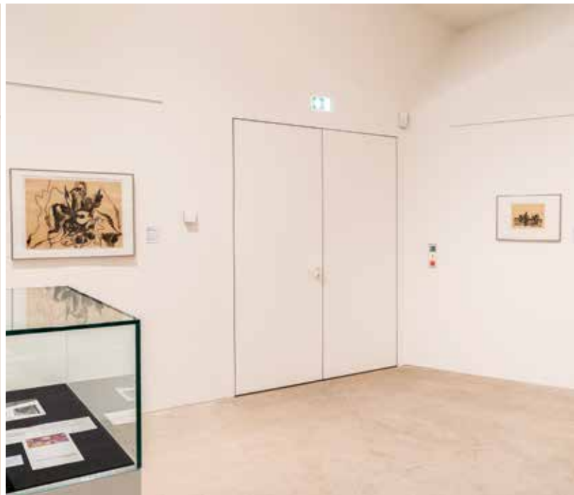
The T30 fire-rated and smoke-tight doors blend seamlessly into the wall.
