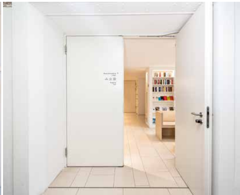
A double-leaf T90 fire-rated and smoke-tight door connects the old and new buildings.
